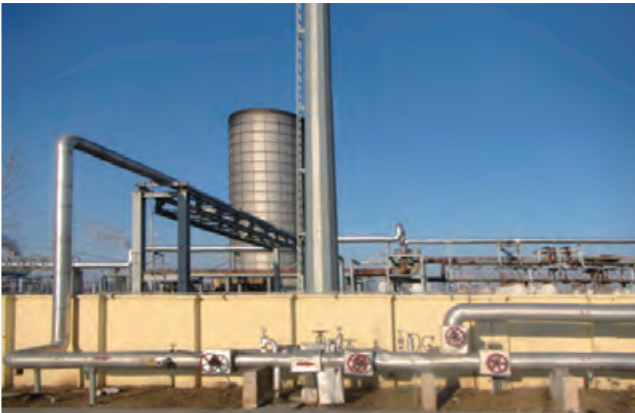
The pipelines for purchased steam
