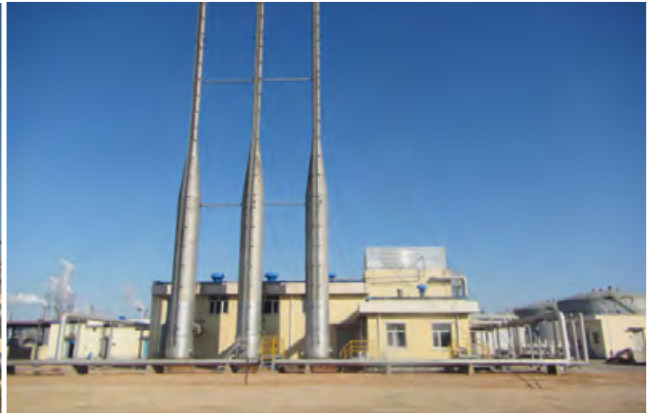
The 3 out of service oil boilers
